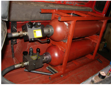
Fig. 9 The accumulators battery
