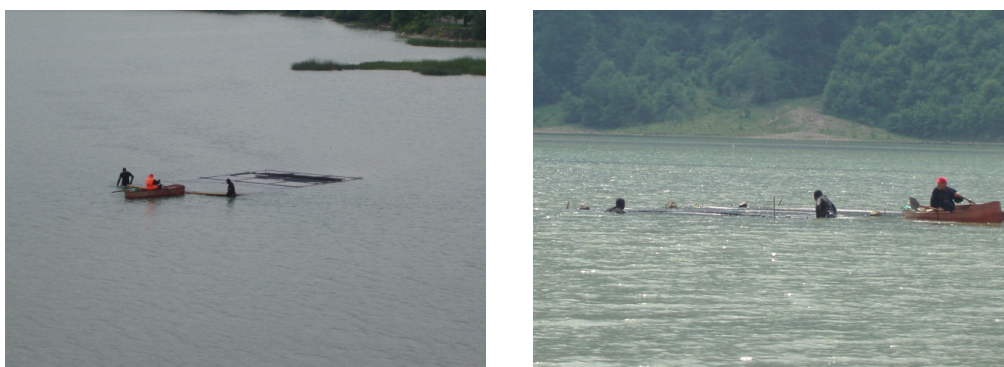
Fig. 5. Images during barriers anchoring
