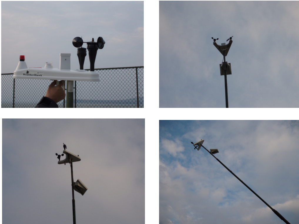
Fig. 2. Images during assembling and installation of monitoring weather station
