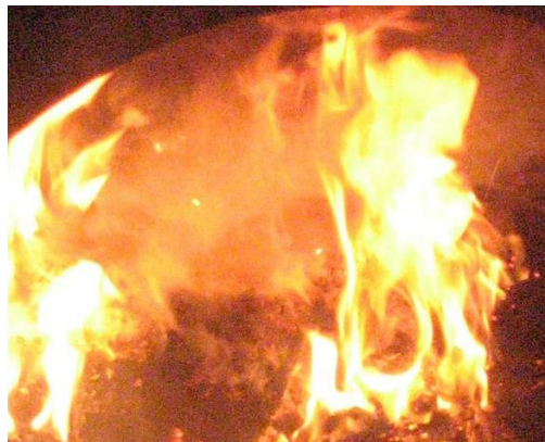
Fig.2. The flame in the 55 kW boiler furnace
