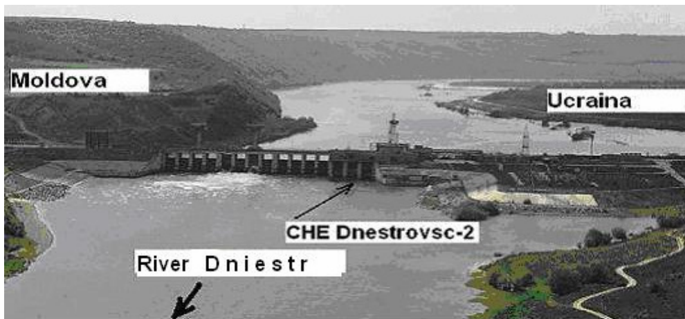
Fig.4.CHE Dnestrovsc-2 (River Dniestr) power plant of 15-40 MW, (MD-UA)
