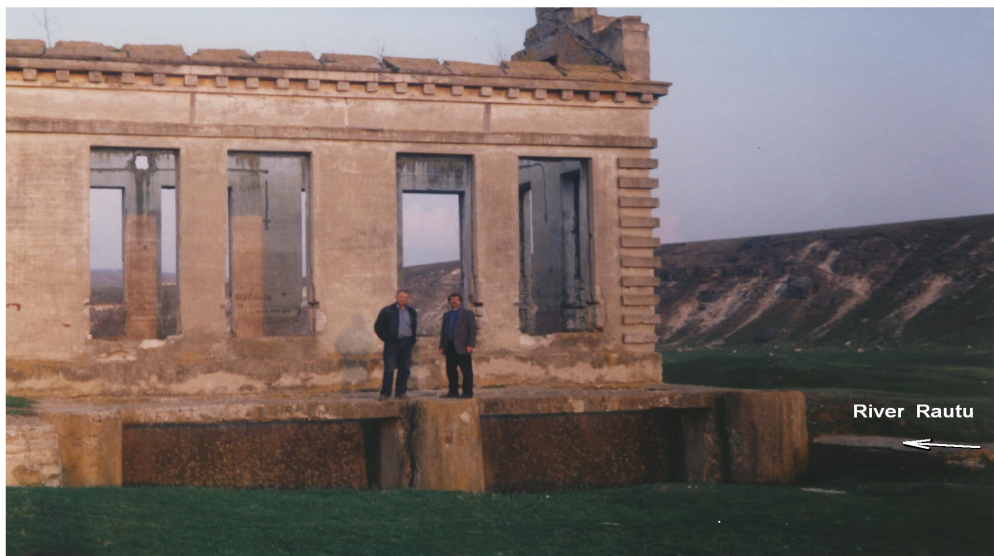
Fig.2. Hydroelectric Power Plant Piatra-Jeloboc on the Raut River (1953)
