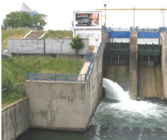
Fig. 4. The photo taken on the actual Ciurel-dam near-by the Polytechnic University of Bucharest, ready to admit on the left side, the closed plant MHPP in question, rated 3 \cdot 100 kW, as installed power.
