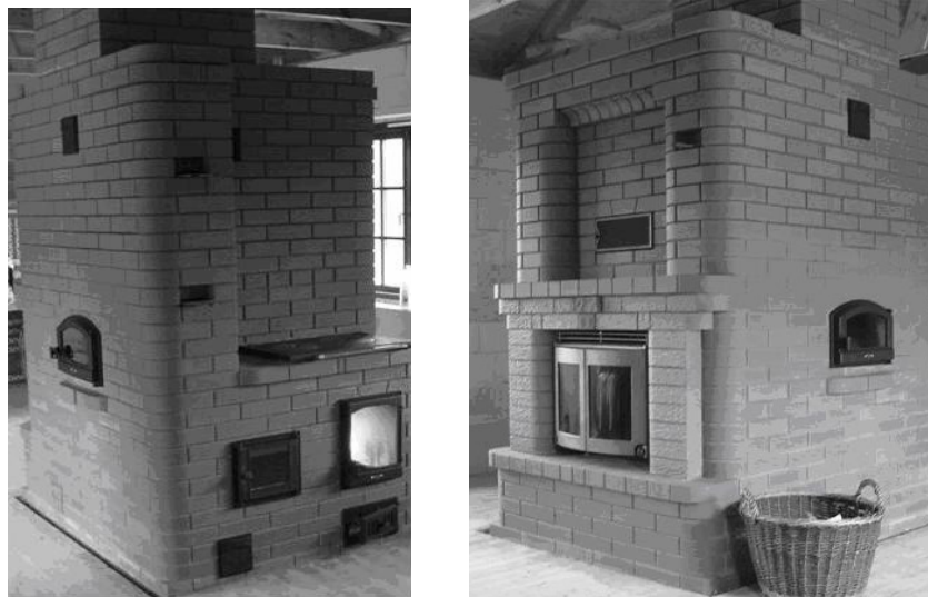
Fig. 1. Multifunctional stove built by the principle of “free gas movement” (Kuznetsov).
