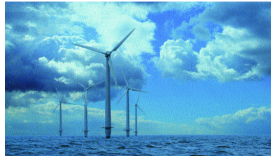
Fig. 3. An offshore wind farm.
