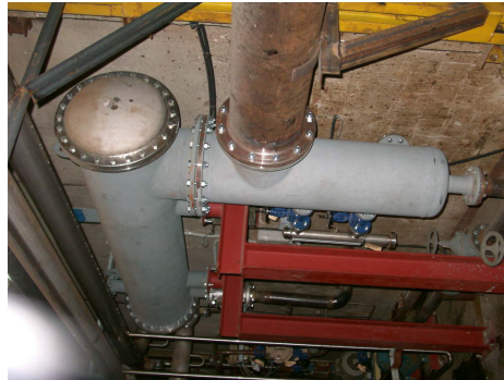
Figure 6 Steam/condensate system of the paper machine [3]
