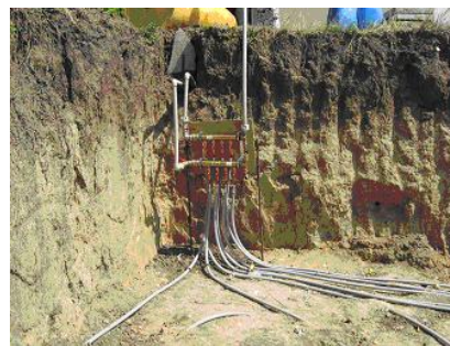
Fig 3. Heat pump. Source distribution system.
