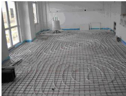
Fig 2. Floor heating system. Polystyrene sheet.
